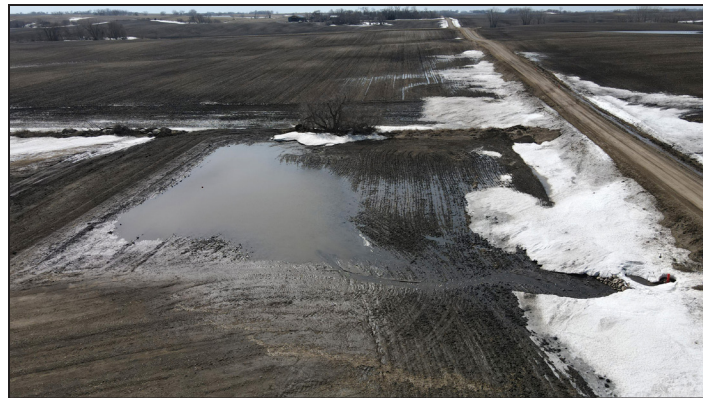
After a sudden warmup followed heavy snows, a water and sediment control basin worked as designed in spring 2023 in a field Mark Thompson farms in the East Branch Chippewa River watershed. Photo Credit: Andy Albertsen, Swift County SWCD
