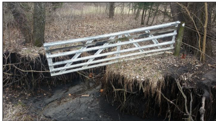
Top: A modified rock weir armored with rock and underlain with erosion-control materials is designed to hold water, curb erosion and stabilize the banks of Judicial Ditch 9. Before the Clean Water Fund-backed project was installed, erosion carved a 50-foot-long, 8-foot-wide gully to Pickerel Lake. Above: The erosion that caused head-cutting and deposited tons of soil into Pickerel Lake also threatened access to landowners’ property. Photos Courtesy SRRWD
