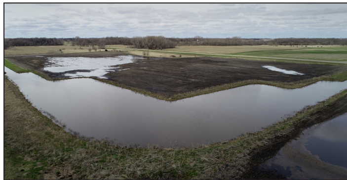
The two-stage ditch constructed as part of the Shell Rock River Watershed District’s Clean Water Fund grant-focused work targeting Pickerel Lake worked as designed after a 5-inch rain. The “steps” are under water.
