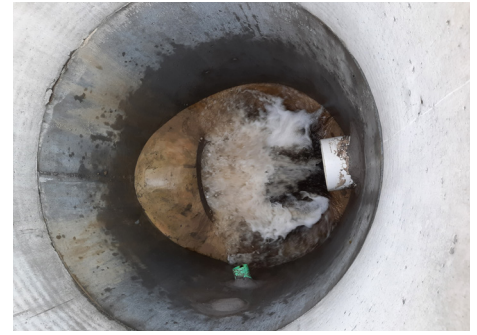
Mower SWCD staff photographed the basin outlet after a late-August rainstorm. Staff notes the project is intended to meter out runoff, allowing sediment to settle out and reducing peak flows that can scour downstream banks. This project will slowly release water over one to three days vs. six to eight hours. Photo Credits: Mower SWCD
