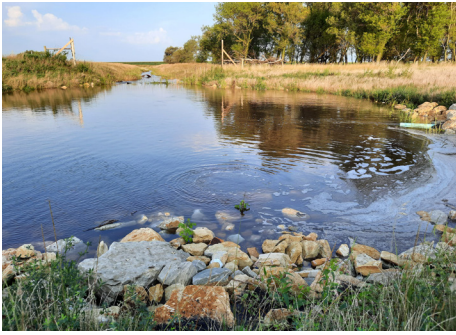
Mower SWCD staff photographed the basin outlet after a late-August rainstorm. Staff notes the project is intended to meter out runoff, allowing sediment to settle out and reducing peak flows that can scour downstream banks. This project will slowly release water over one to three days vs. six to eight hours. Photo Credits: Mower SWCD
