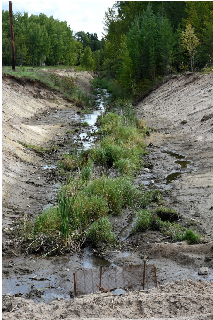
The Lake Irving ditch is being re-meandered to look and function more like a stream. It’s part of the Beltrami SWCD’s Clean Water Fund-backed stormwater treatment project, which is designed to benefit nutrient-impaired Lake Irving and estimated to keep 233 pounds of phosphorus out of the lake each year.
