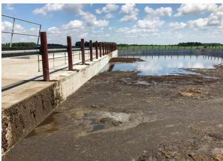
Left: The fencing Ben and Jay Currier installed along the edge of the pit can be raised and lowered. Having two points to scrape manure into the pit gives them an option if buildup occurs during winter freezes. The 1.4 million-gallon design allows for increased volume due to rainfall. Middle: The previous storage area, left of the open barn door, held a week's worth of manure. Right: Grooves in the concrete increase traction.
