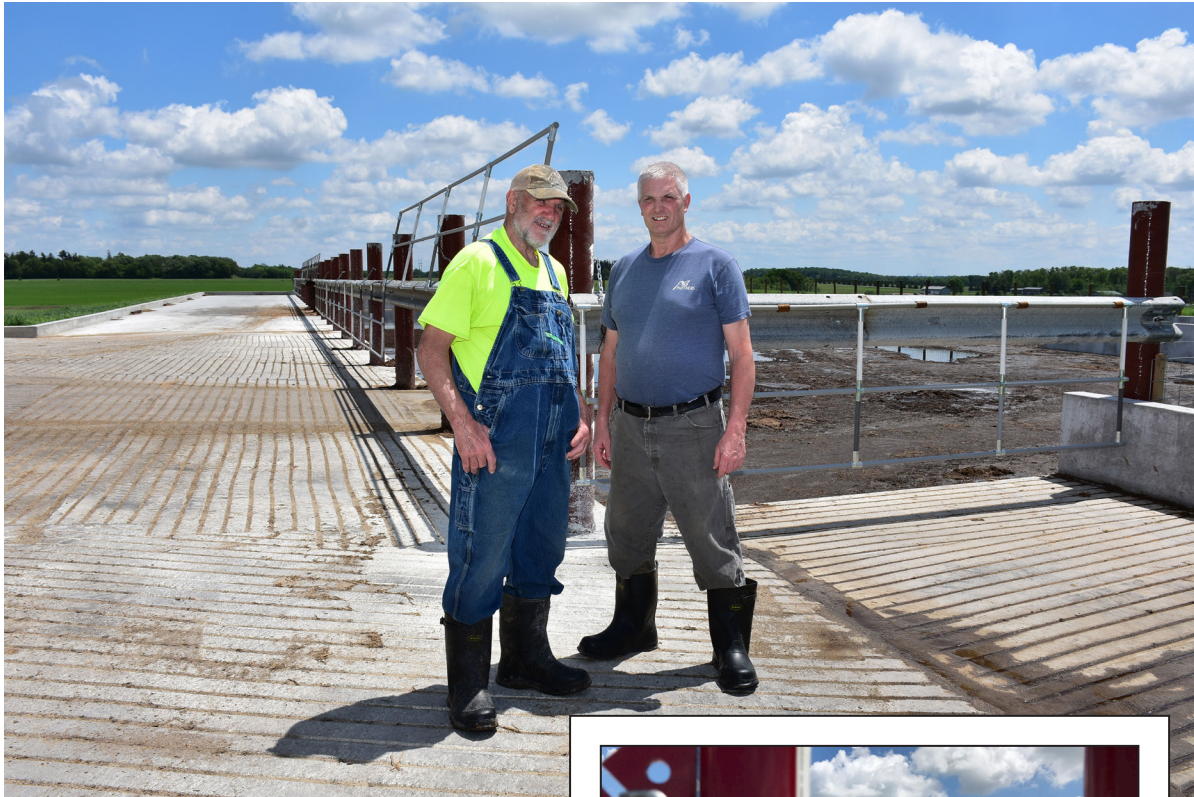
Top: By May, the manure storage facility on the Currier brothers' Mantorville Township dairy farm held seven months' worth of manure. It's built for 12 months of storage, with extra capacity in case of emergency. The cow yard slopes to the pit. Jay (left) and Ben Currier previously had one week of storage. The facility was installed with assistance from the Lower Mississippi River Feedlot Management in Minnesota Regional Conservation Partnership Project, which is funded jointly by the USDA's NRCS and by BWSR. Bottom: A ramp allows for easy access to clean out the pit. Photo Credits: Ann Wessel, BWSR
