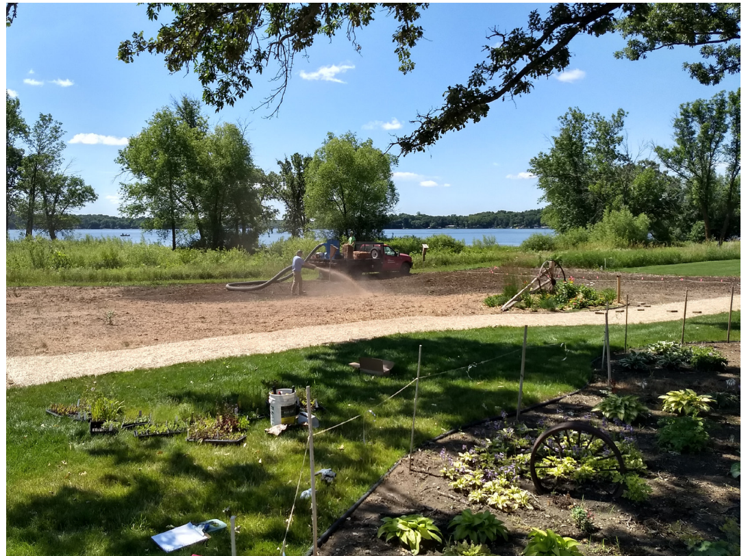
A landscaping contractor applies a layer of straw to protect this recently seeded Sherburne County pollinator meadow from erosion.
