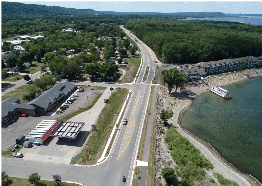
Before the stormwater basins were installed on the north end of Lake City, urban runoff from 15 acres drained directly into Lake Pepin and a nearby creek. Lake Pepin is a 21-mile-long widening of the Mississippi River. When it became apparent during construction that one of the basins was close to a city water main, city staff located the pipe, which was then insulated to avoid freezing in the winter.
