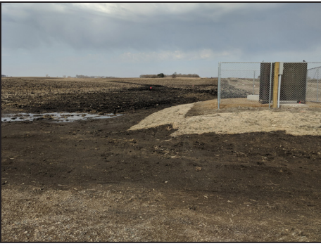
From left: On Stan Gorecki's 60-acre RIM easement, Area II helped to design and install a pump station that lifts water 12 feet from tile that's part of Lincoln County Ditch 37. Water pumped by the lift station from the tile first enters this basin, seen after snowmelt in April 2018. Raising a township road made it possible to increase floodwater storage on Steve Snyder's land to 61 acre-feet. Photo Credits: Area II Minnesota River Basin Projects
