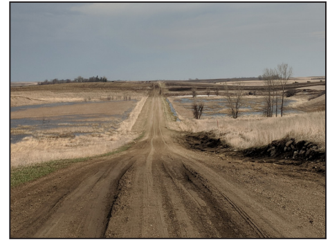
From left: On Stan Gorecki's 60-acre RIM easement, Area II helped to design and install a pump station that lifts water 12 feet from tile that's part of Lincoln County Ditch 37. Water pumped by the lift station from the tile first enters this basin, seen after snowmelt in April 2018. Raising a township road made it possible to increase floodwater storage on Steve Snyder's land to 61 acre-feet. Photo Credits: Area II Minnesota River Basin Projects
