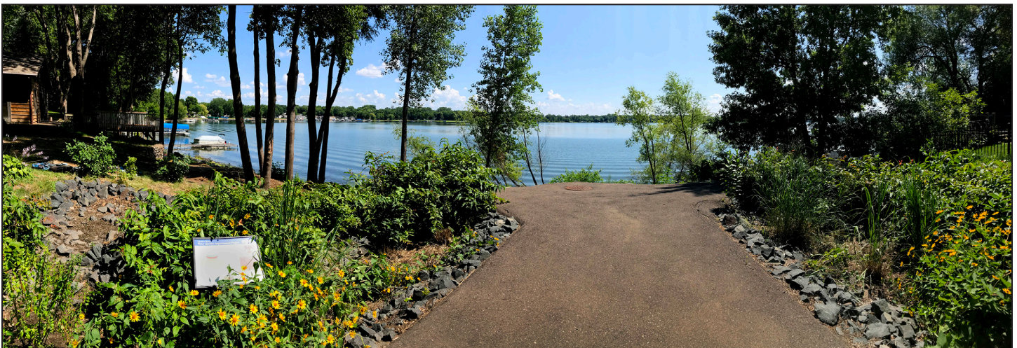
In Lindstrom, new or rebuilt city streets are made narrower when possible — a strategy that reduces stormwater runoff and cuts city maintenance costs. Linden Street was made narrower where it dead-ends at South Lindstrom Lake. It’s flanked by a stormwater treatment system that includes rain gardens.
