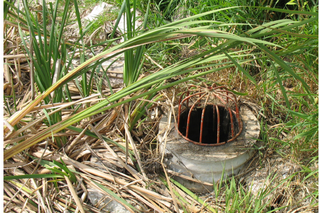
Figure 6.10 Drop inlet structure for wetland outlet
