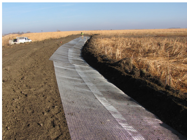
Figure 6.8 Installing fence to prevent muskrat burrows in an embankment
