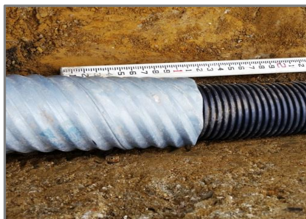
Figure 5. Metal Sleeve Placed over Tile at Outlet (pre-grouting)
