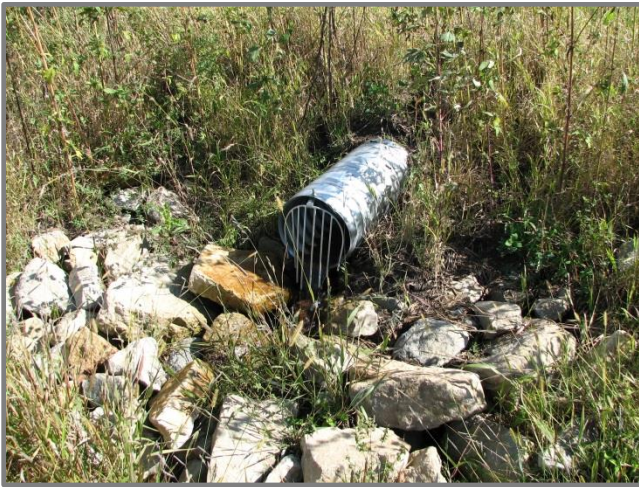
Figure 6. Riprap Protection at Tile Outlet
