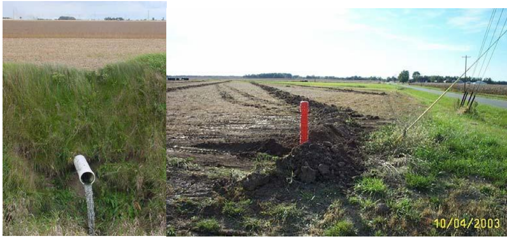
Figure 14: Tile Outlet into Drainage Ditch (left photo) and Perforated Tile Riser Inlet (right photo)
