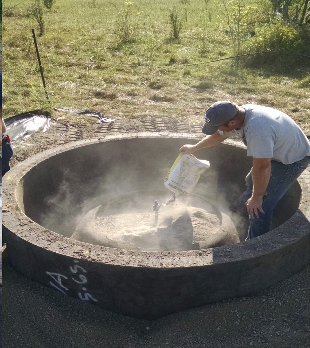
Summer water tank installation. Evolved to 14 tanks and a total of 18,400 feet of waterline over all managed pastures.
